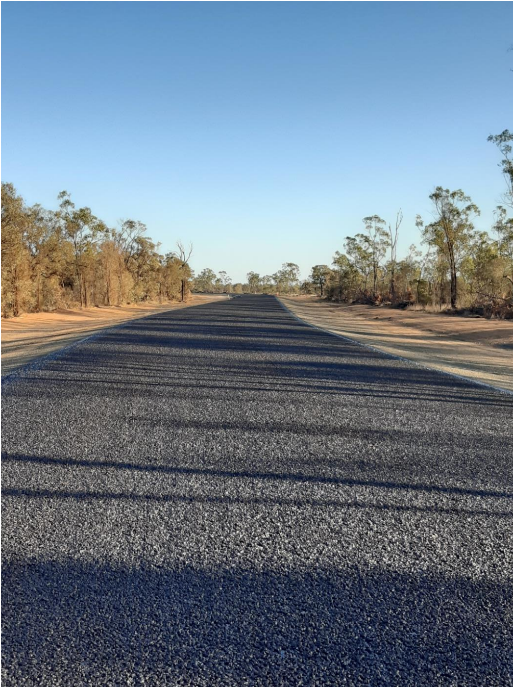
CW 212888 Eaglefield Pave & Seal – Bottom Coat Seal Works – completed
