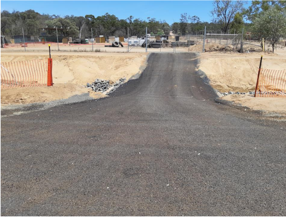
CW182485 Sarchedon Drive – Access driveways – completed
