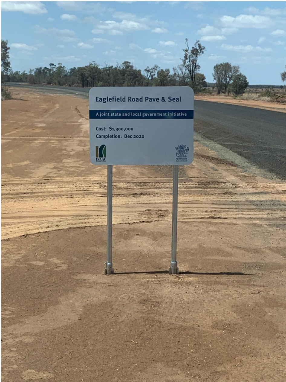
CW 212888 Eaglefield Pave & Seal – Project Sign Installation
