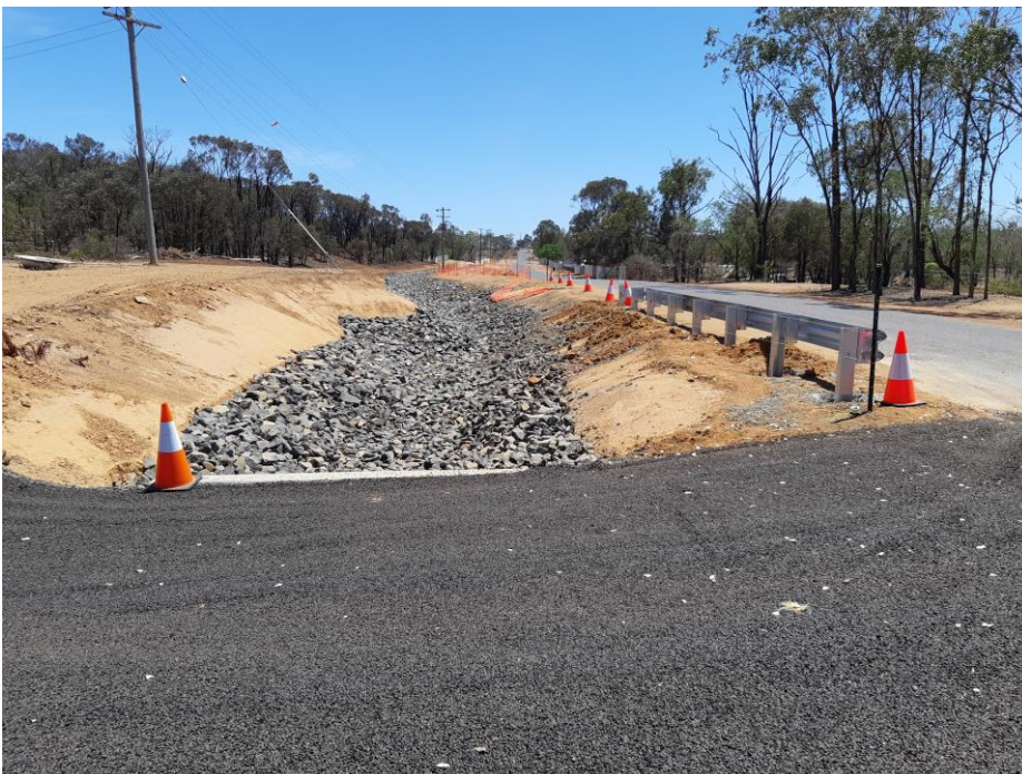
CW182485 Sarchedon Drive – Drainage works – completed
