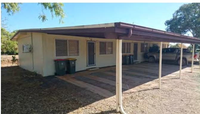
6 Wilangi Street Before
