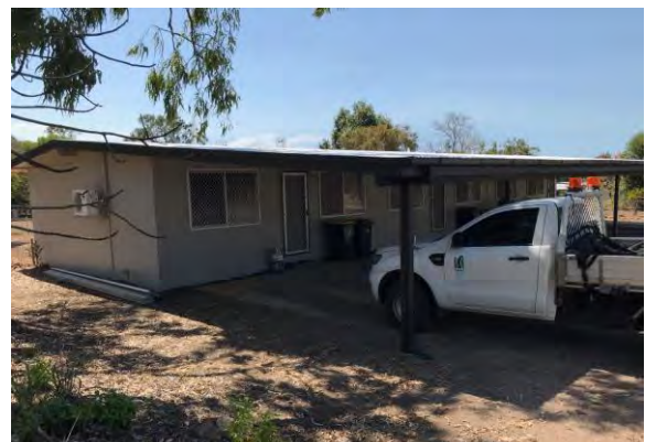
6 Wilangi Street After
