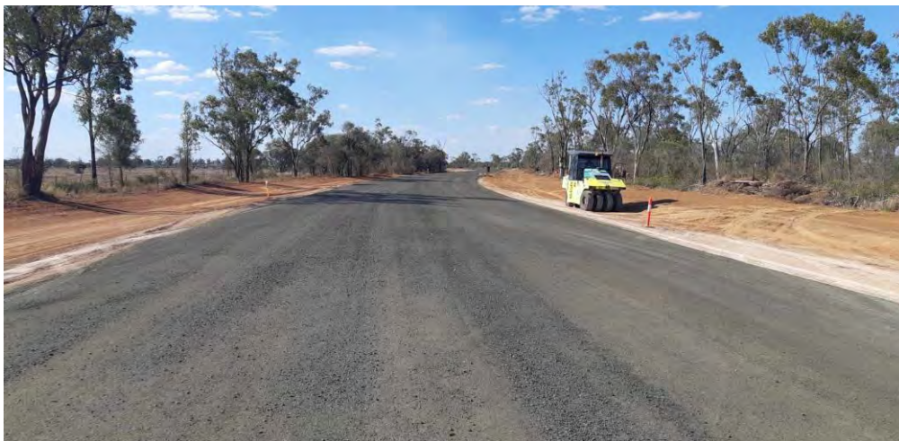
Eaglefield Pave & Seal – Pavement Works
