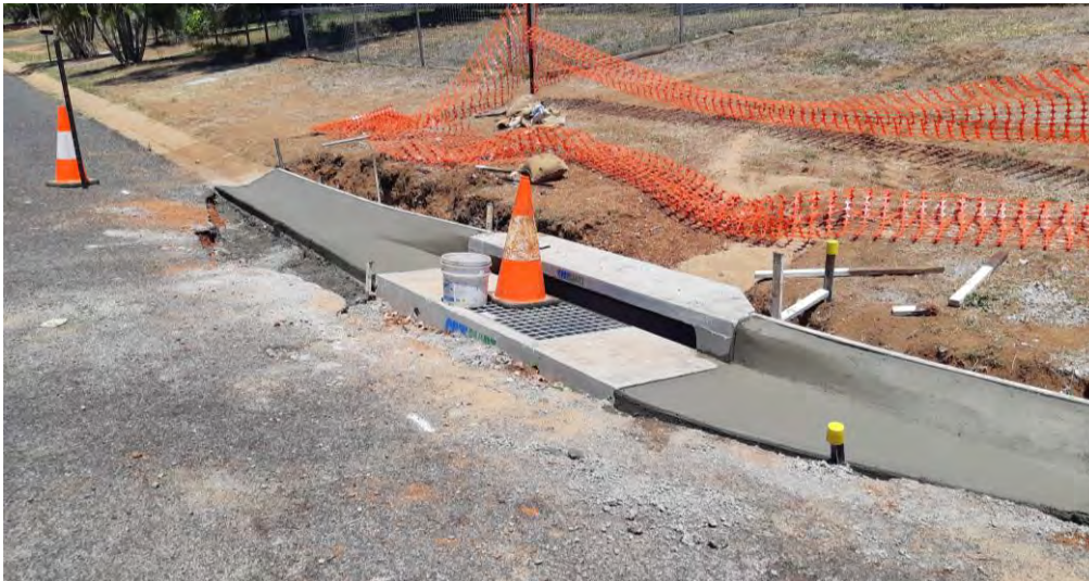
Urban stormwater renewal in Clermont complete.
