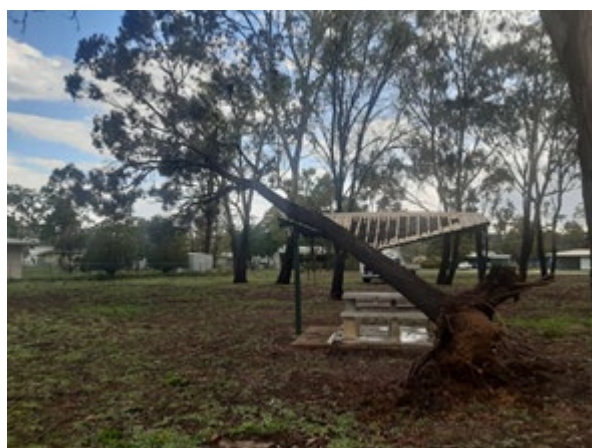
Curllew Park storm damage to shelter
