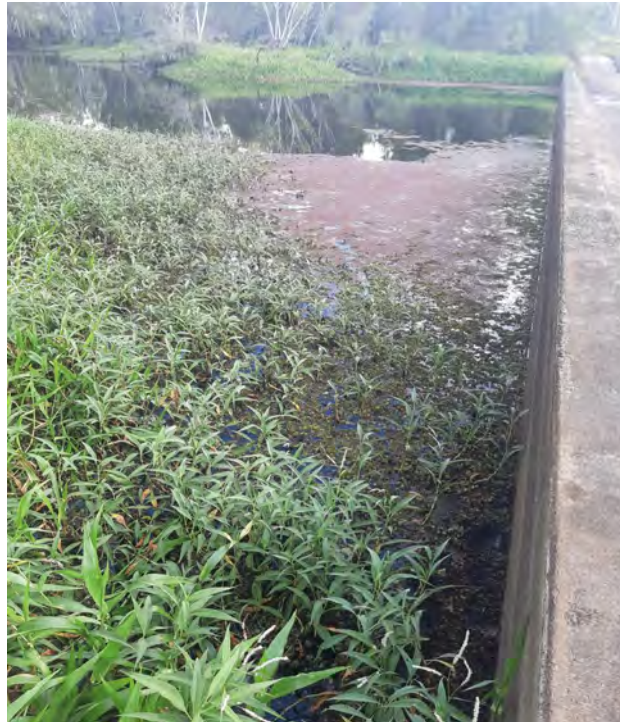
St Lawrence Weir as of 25/02/2020
