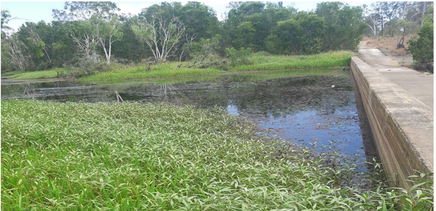
St Lawrence Weir as at 29 October 2021
