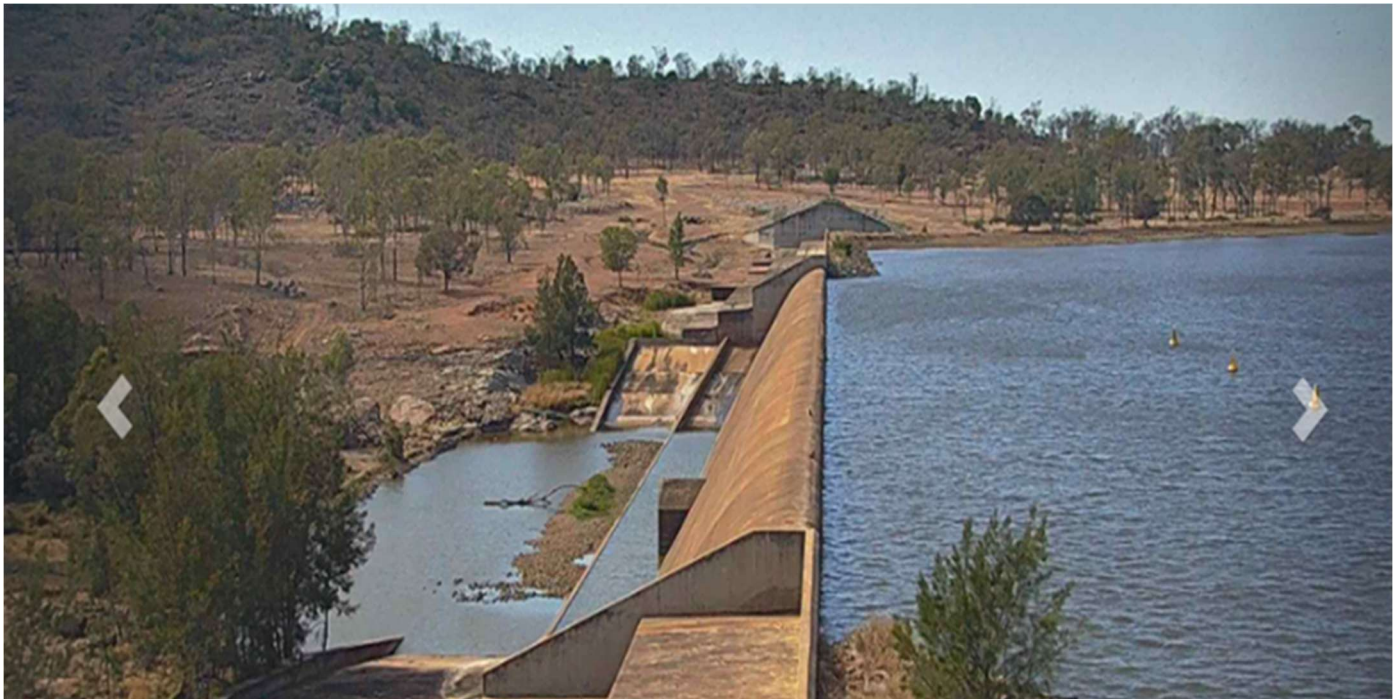
Theresa Creek Dam Wall as at 31 October 2021
