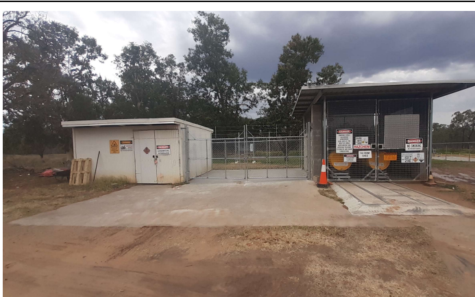
Figure 1 – Newly constructed cylinder storage area
