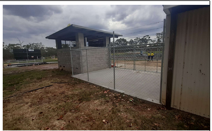
Figure 2 – Newly constructed cylinder storage area
