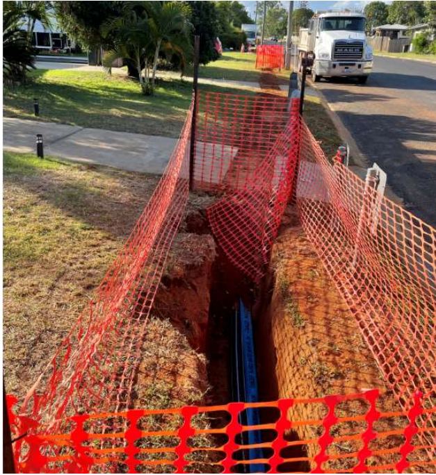
Figure 3 – Installation of new water main
