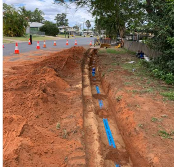
Figure 4 - Installation of new water main
