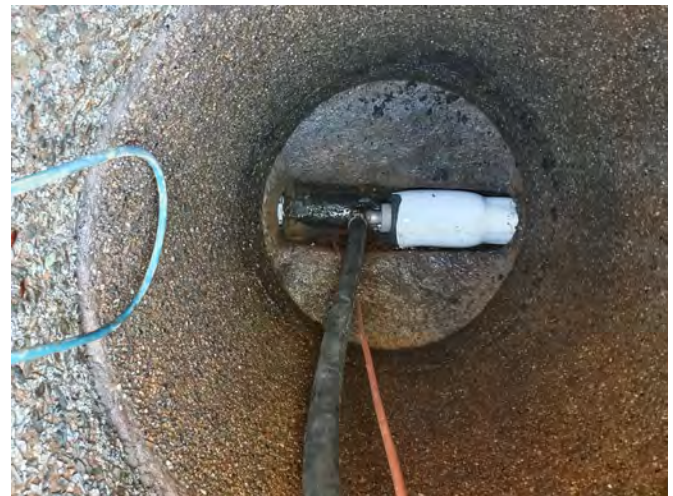
Figure 2 – Low pressure expanding of 225mm fold & form liner Middlemount
