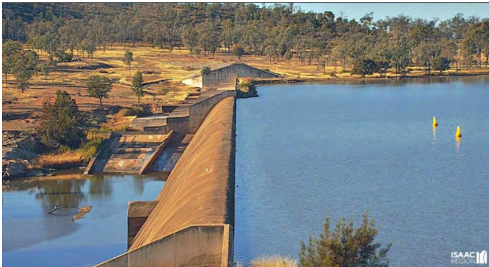
Theresa Creek Dam Wall as at 30 June 2021
