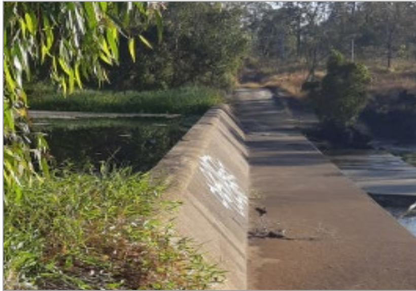
St Lawrence Weir as at 30 July 2021
