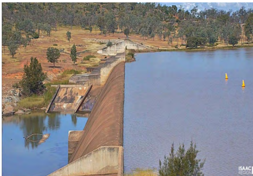
Theresa Creek Dam Wall 30 April 2021
