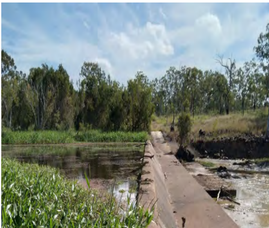
St Lawrence Weir as of 28 April 2020
