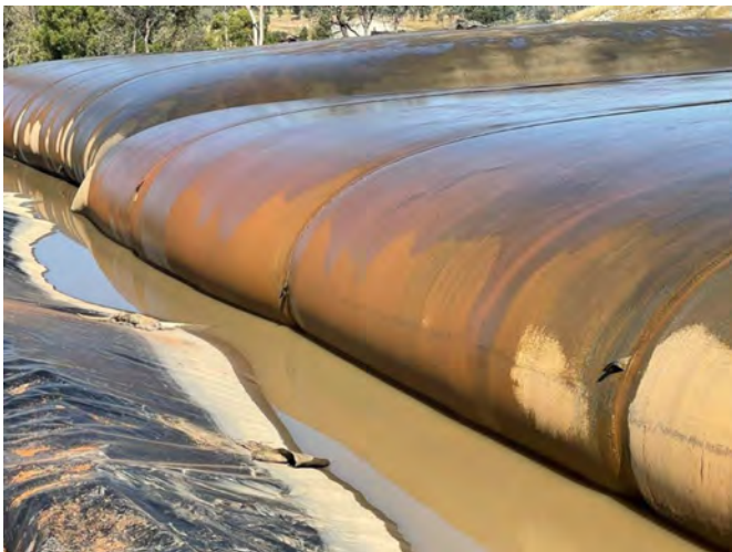
Figure 1- Showing the geotubes with some areas starting to dry out
