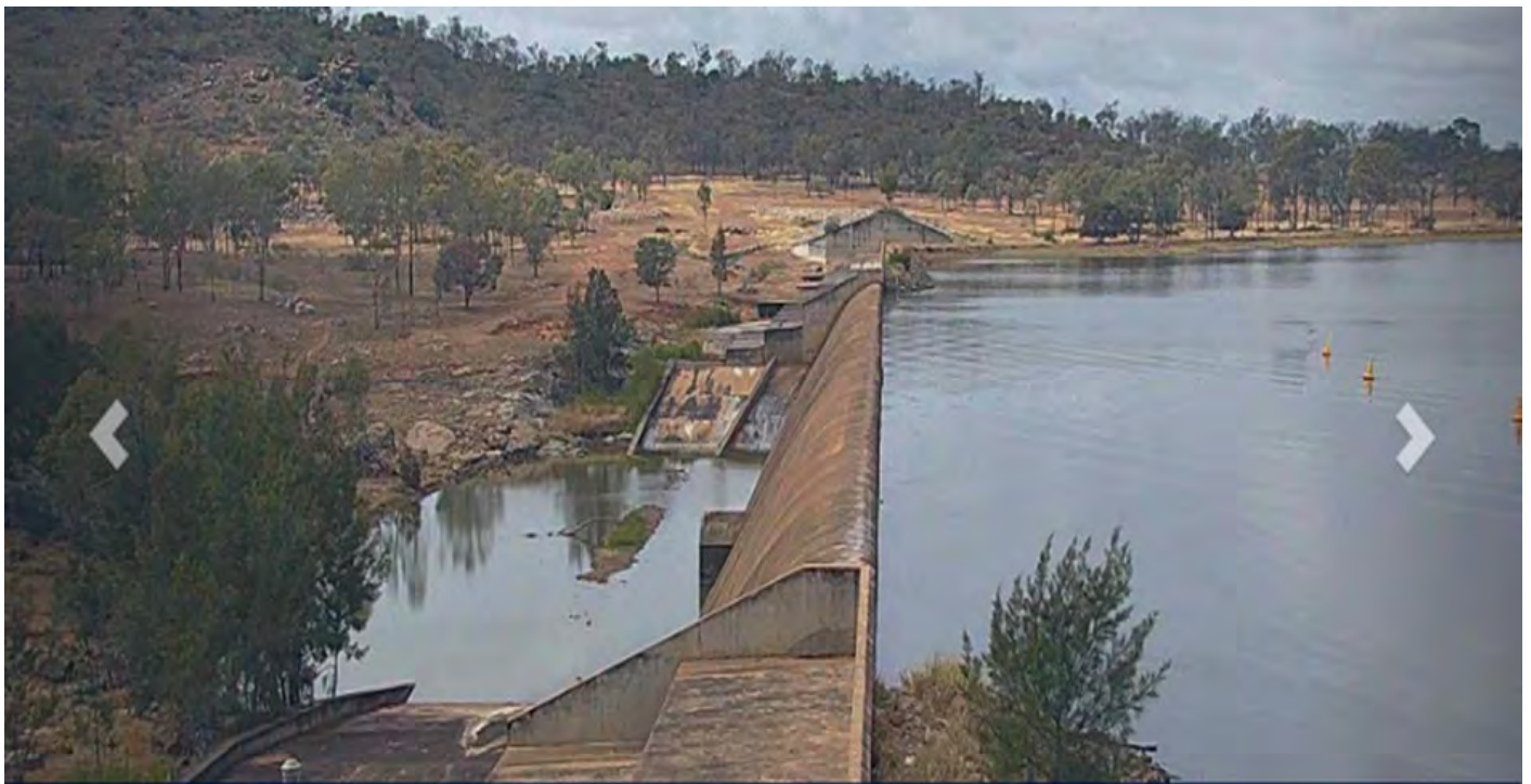
Theresa Creek Dam Wall as at 30 September 2021
