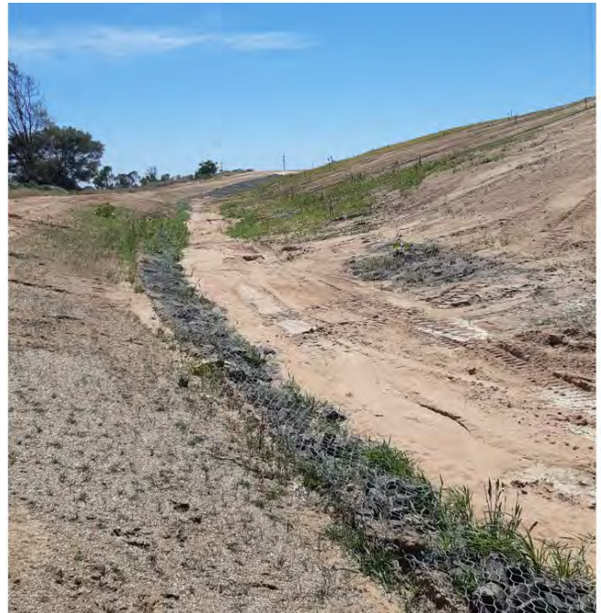
Photo 2 – diversion drain 1 with build of materials
