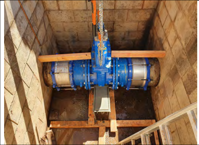
Figure 2 – 375 Valve replacement 3ML inlet
