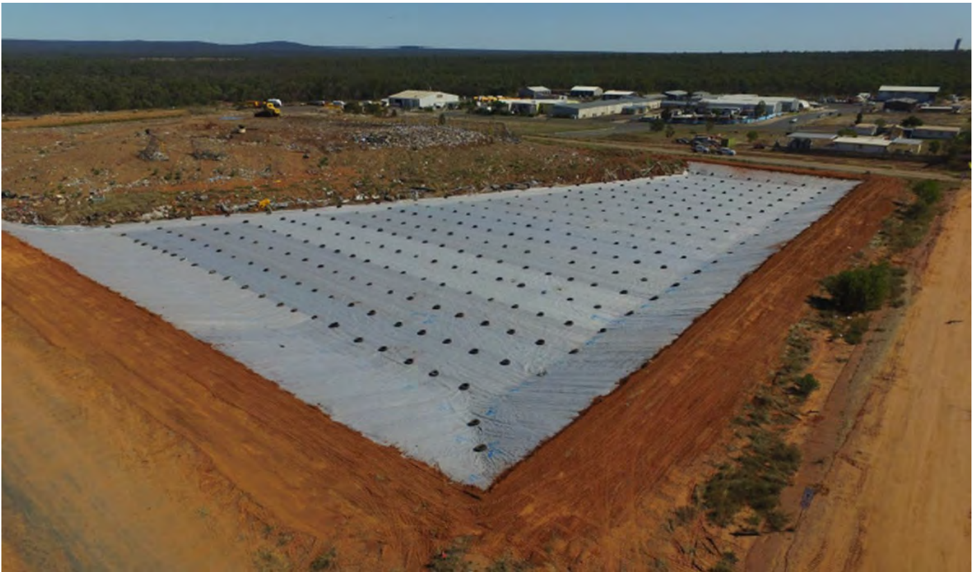
Reinstated Separation Layer in place, Subcell B, Moranbah Landfill Cell 1, June 2021
