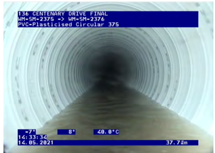
Figure 4 – Completed spiral wound reline of 375 AC main MMT
