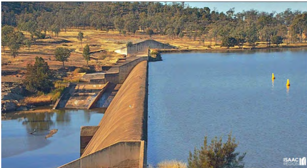
Theresa Creek Dam Wall as at 30 June 2021
