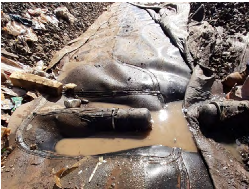
Drainage systems in Subcell A (left) and B (right) prior to connection
