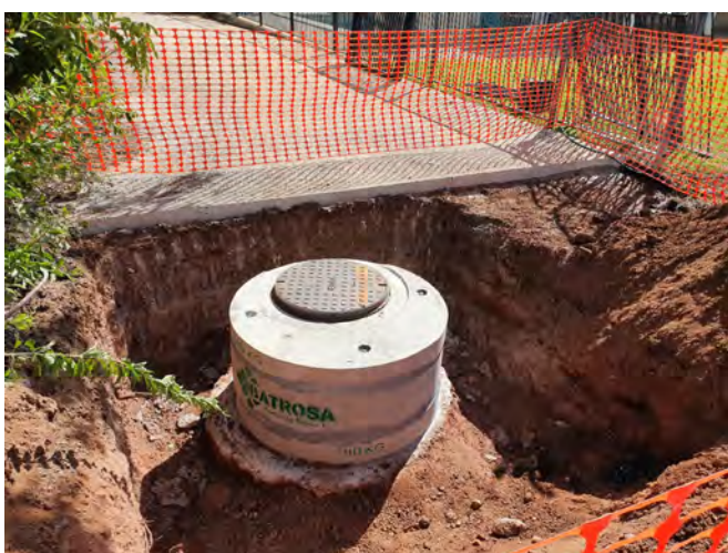
Figure 1 – Image of existing manhole buried below concrete driveway in Clermont
