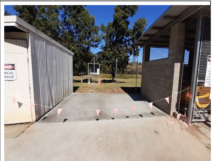
Figure 2 – New slab for storing of gas cylinders
