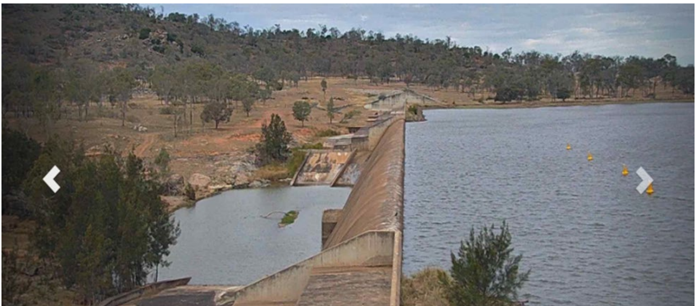
Theresa Creek Dam Wall as at 27 August 2021
