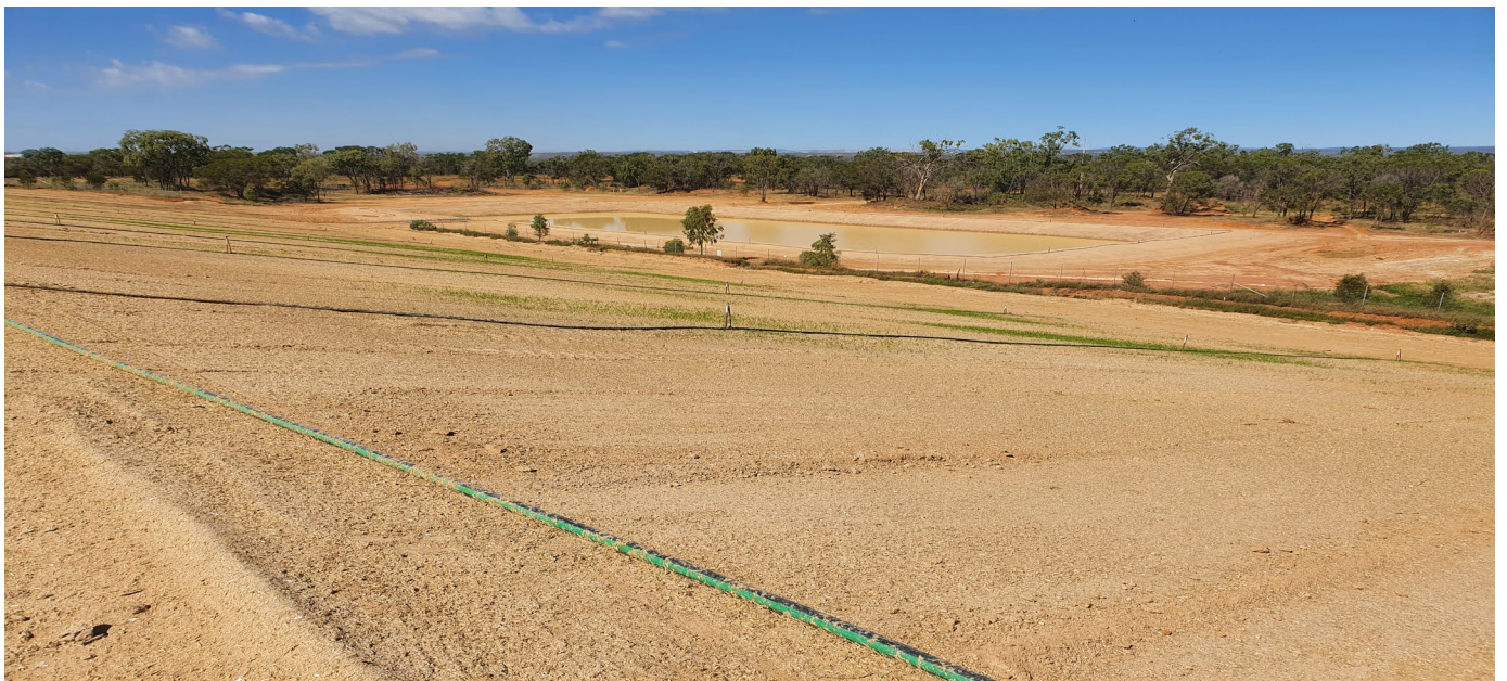
Figure 3 – Side wall of landfill - grass being established
