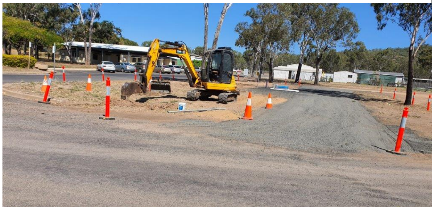
Figure 1 – Initial construction of Middlemount dump point
