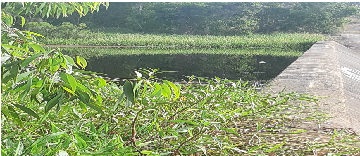
St Lawrence Weir as at 27 August 2021
