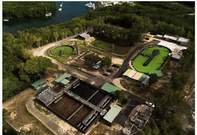
Douglas Shire Council water treatment plant © Douglas Shire Council
