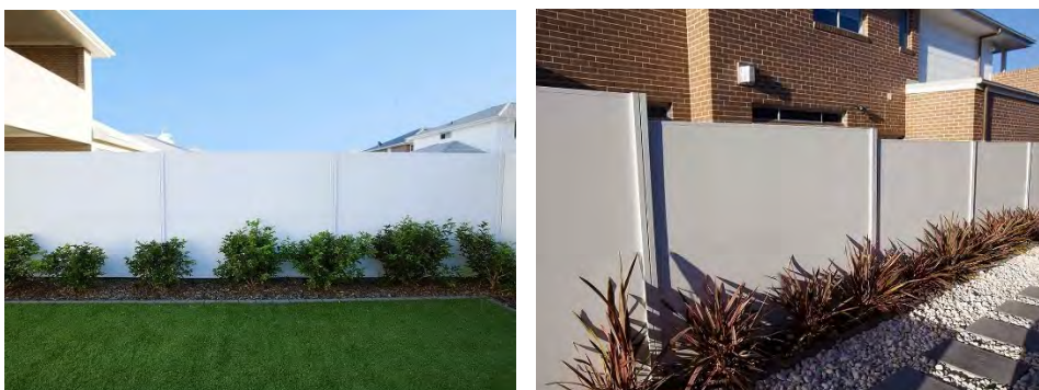
Example of noise attenuation fencing (source: http://www.slimwall.com.au/gallery )
