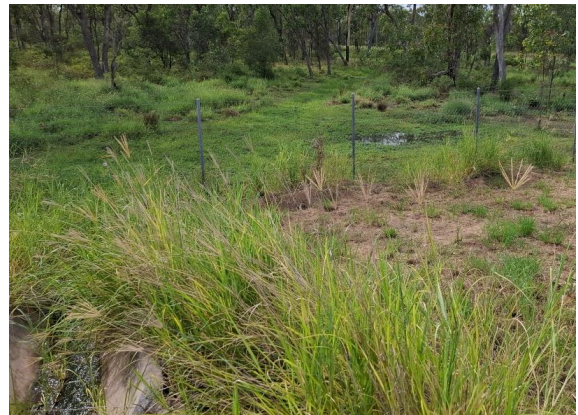
Middlemount Spillway Flow Area
