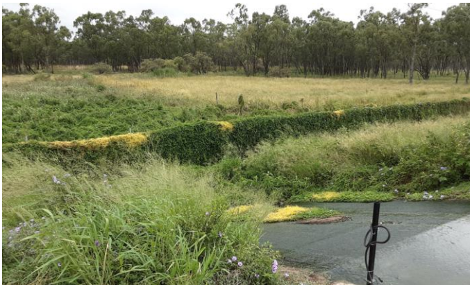
Moranbah Spillway Overtopping
