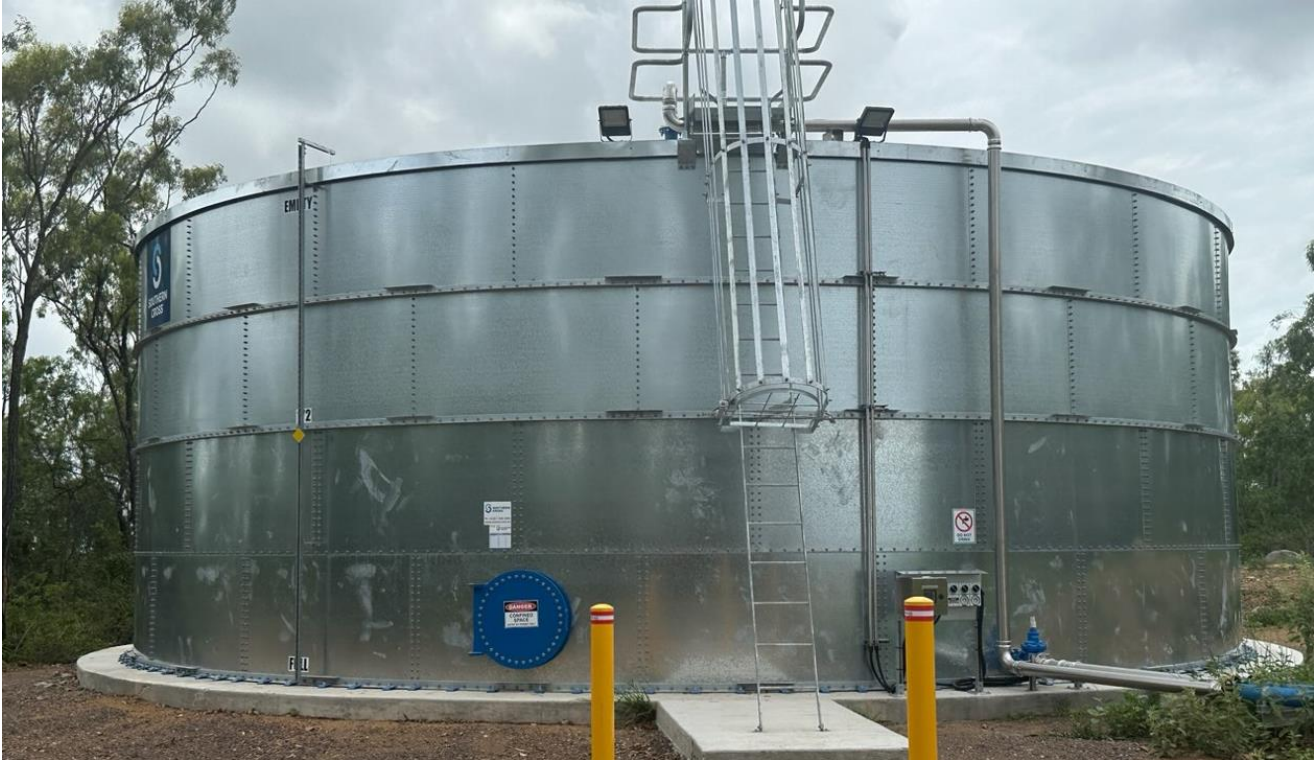
Image 1: St Lawrence Raw Water Tank – Installation Complete
