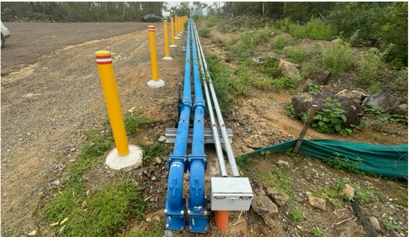
Image 2: St Lawrence Raw Water Main – Installation Complete
