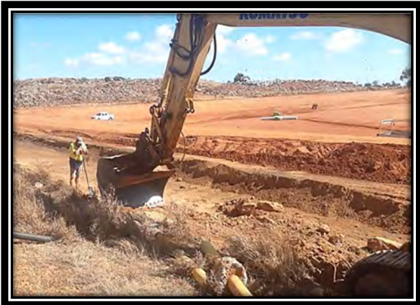
Image 3: Clearing and Excavation in progress
