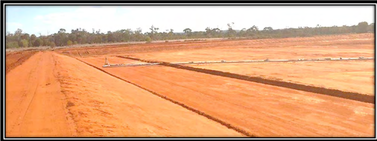
Image 5: Shaping of the bed of the cell is nearly complete
