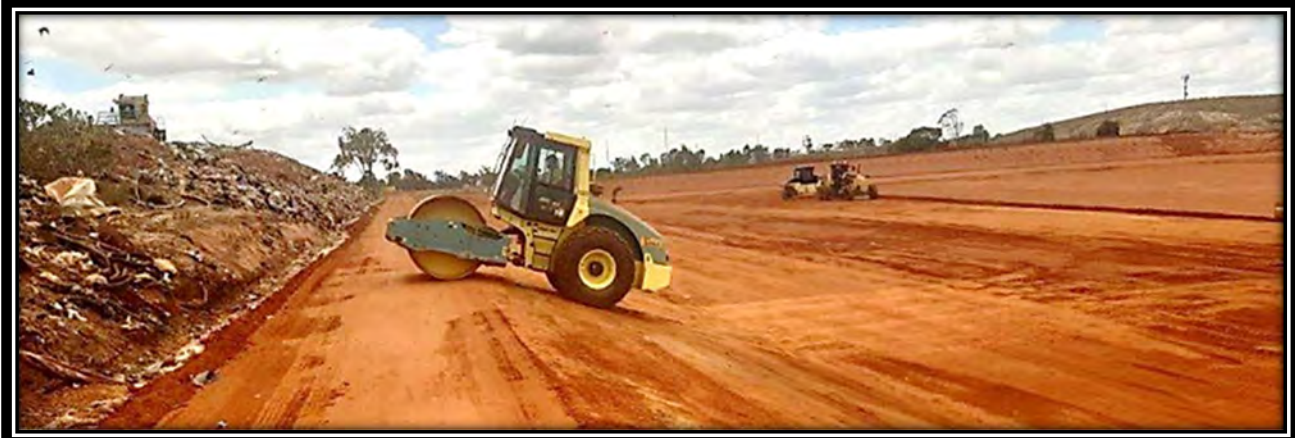
Image 4: Shaping of the bed of the cell
