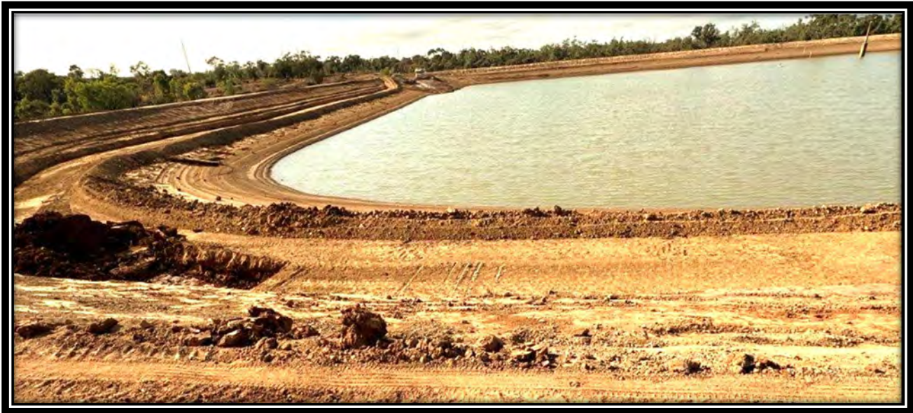
Image 6: Earthworks in progress along the dam
