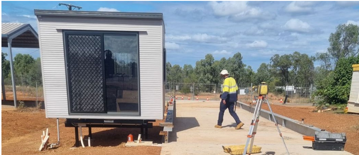
Image 1: Clermont Waste Management Facility Gatehouse Installation in progress
