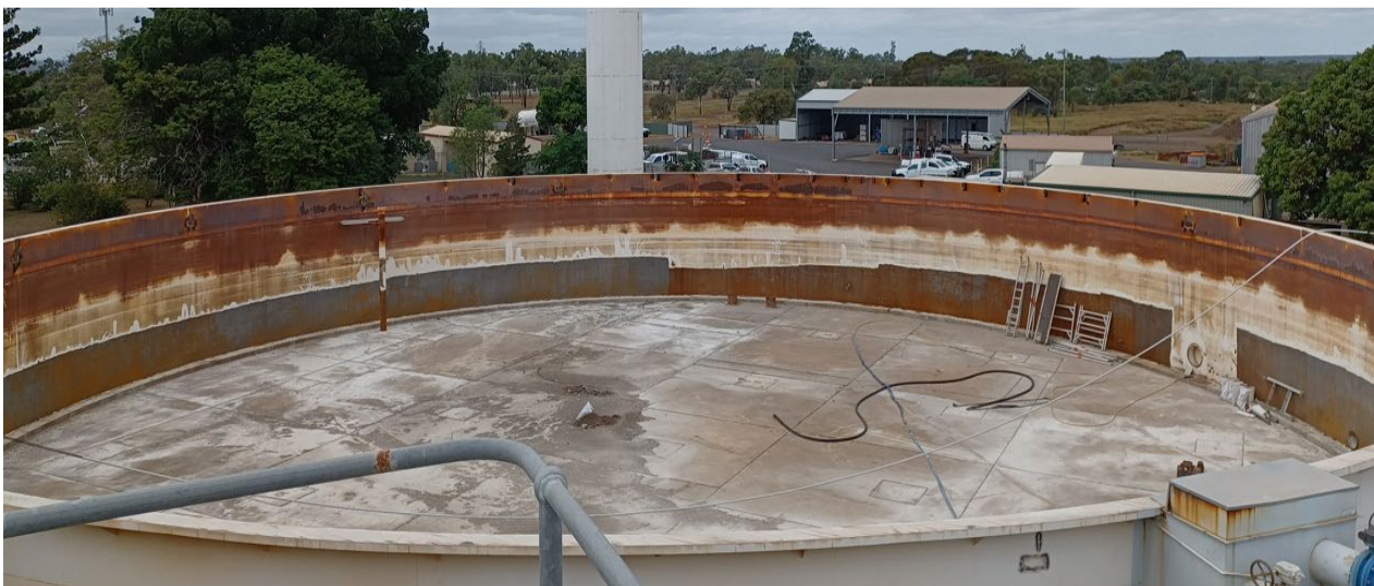
Image 2: Moranbah WTP Roof Replacement - Painting internal wall in progress
