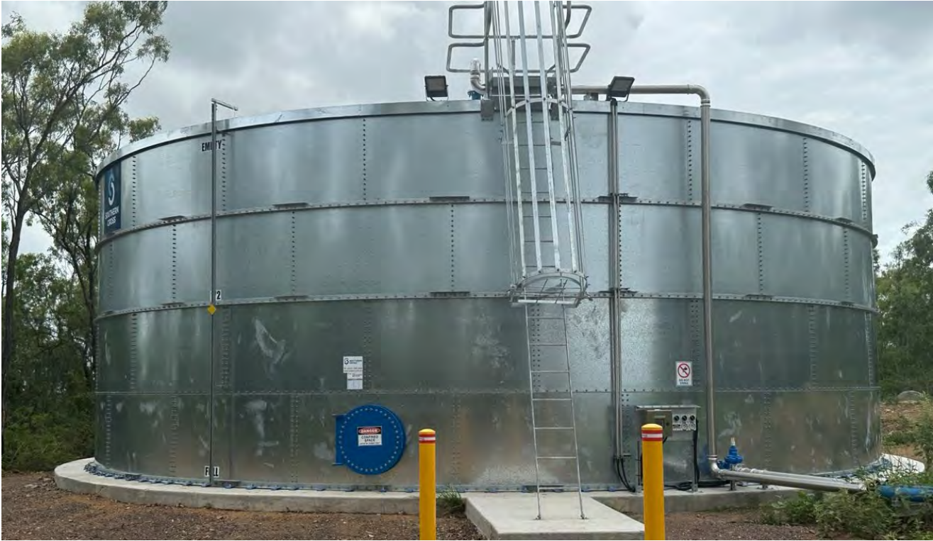
Image 1: St Lawrence Raw Water Tank – Installation Complete
