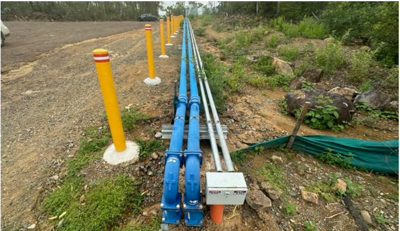
Image 2: St Lawrence Raw Water Main – Installation Complete
