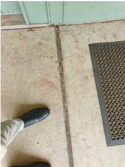
Sealant cracking
