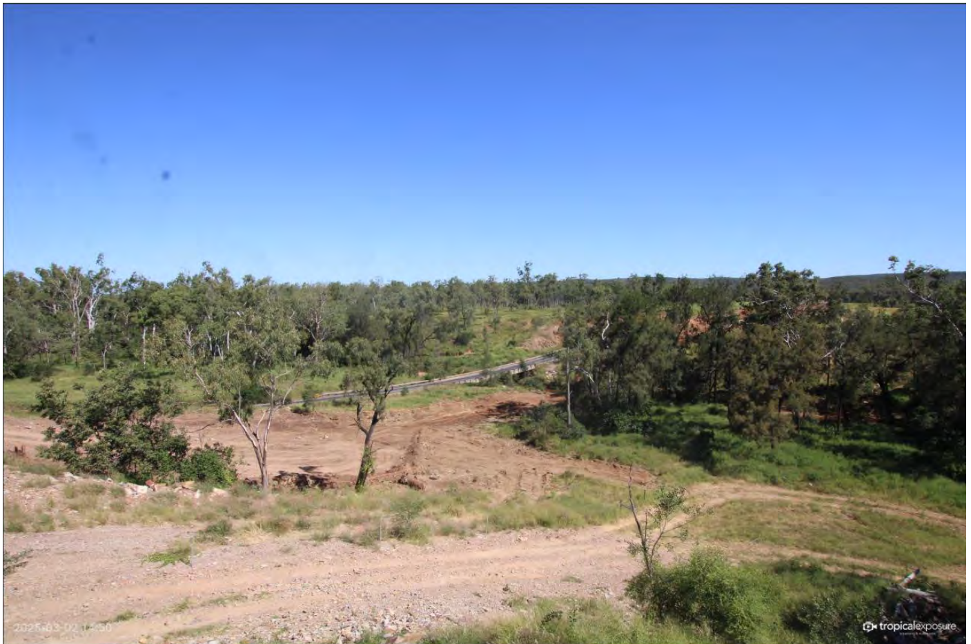
Figure 3: Phillips Creek Bridge Timelapse Camera 2/3/25
