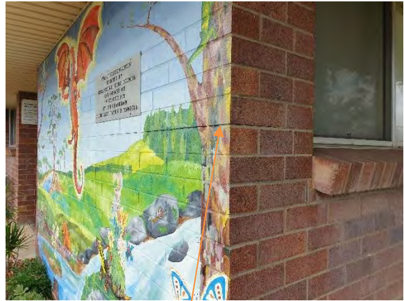
Minor brick cracking
