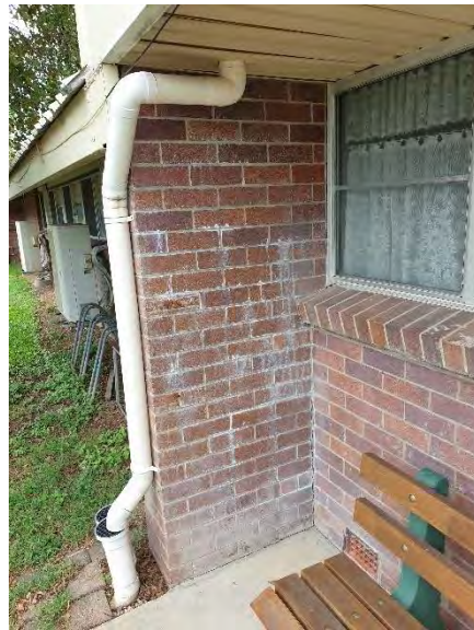
Brick efflorescence
