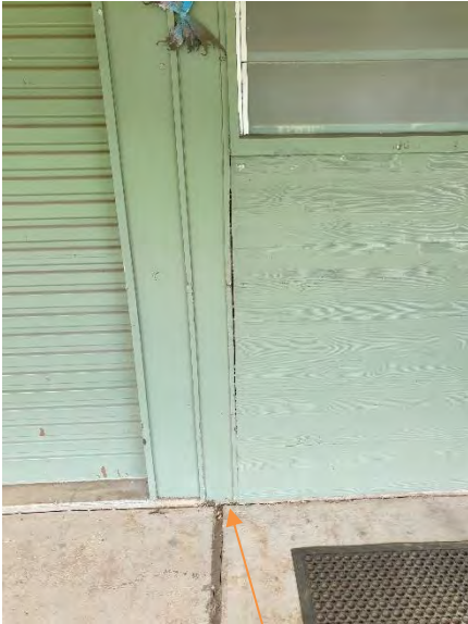
Minor rust at base of steel column
