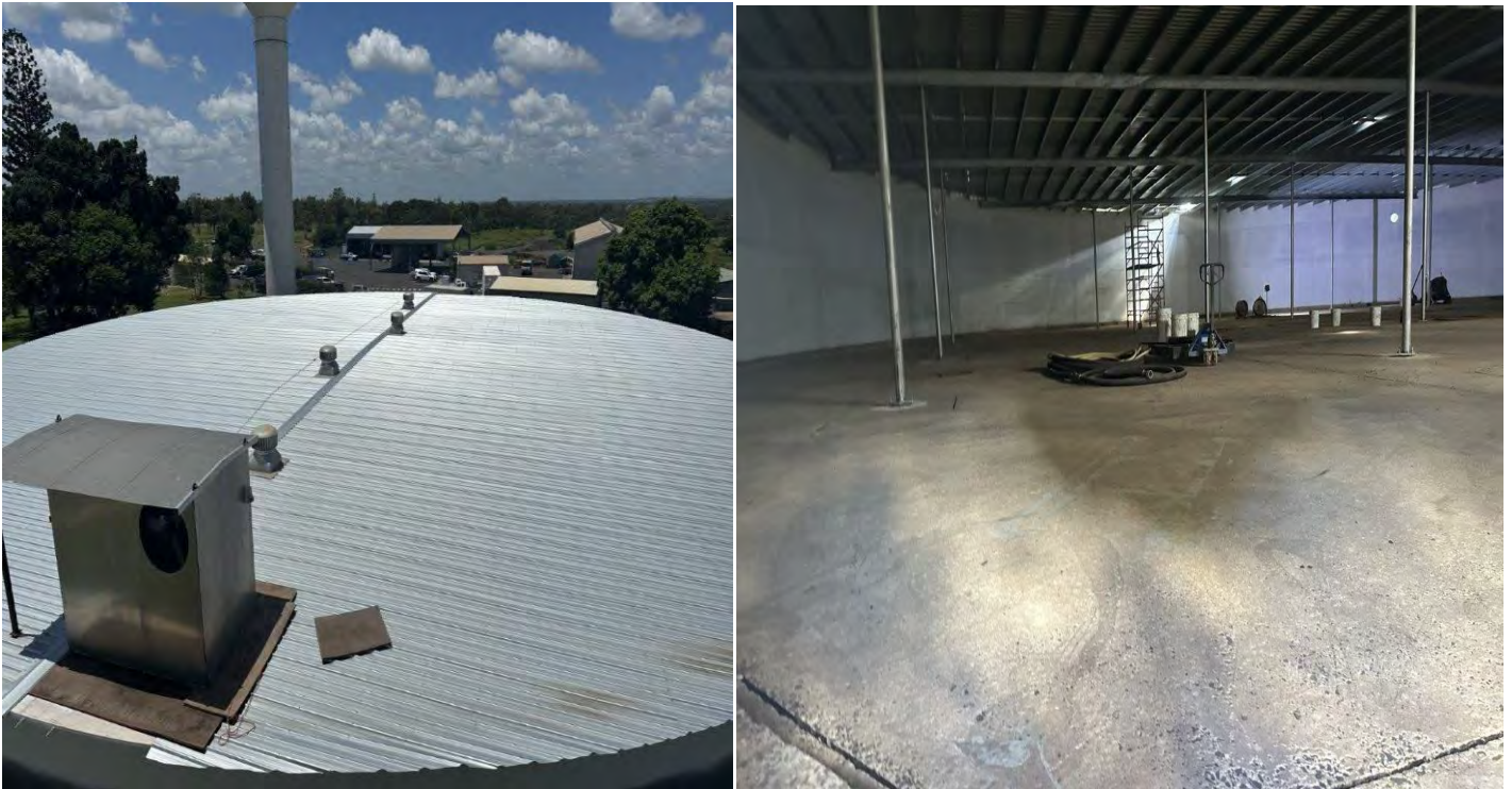
Image 3: Moranbah Water Treatment Plant Roof Replacement – Nearing Completion
