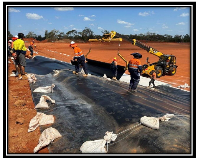
Image 5: Laying Geo-membrane in progress
