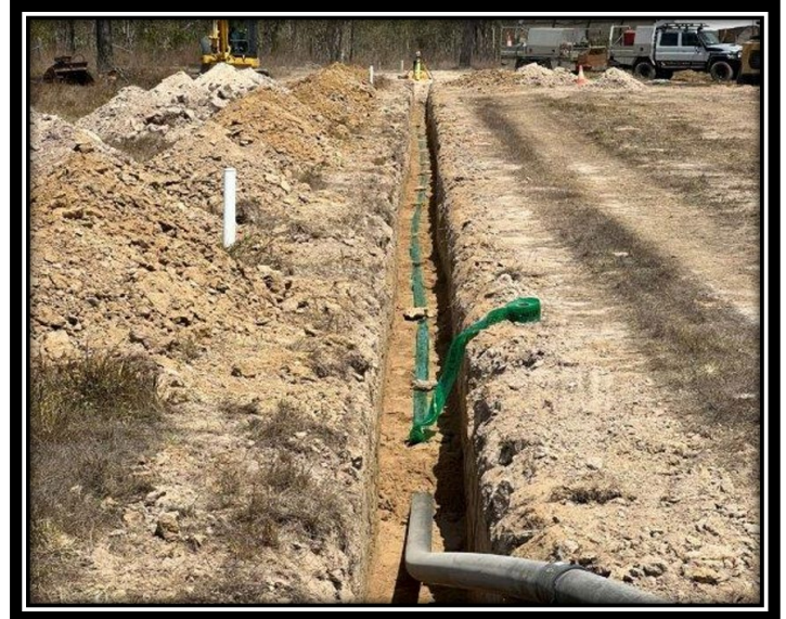
Image 7: Pipe laying in progress
