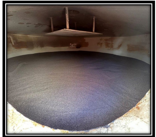
Image 2: Filter media replacement complete
