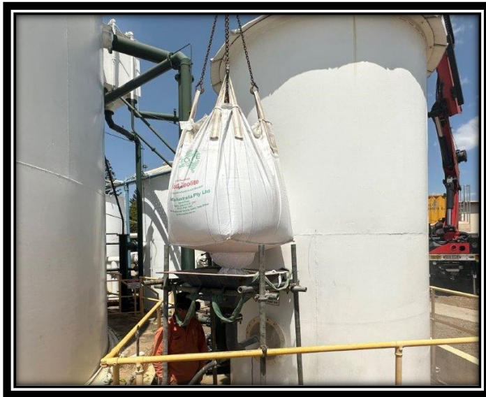
Image 1: Filter Media placement in progress
