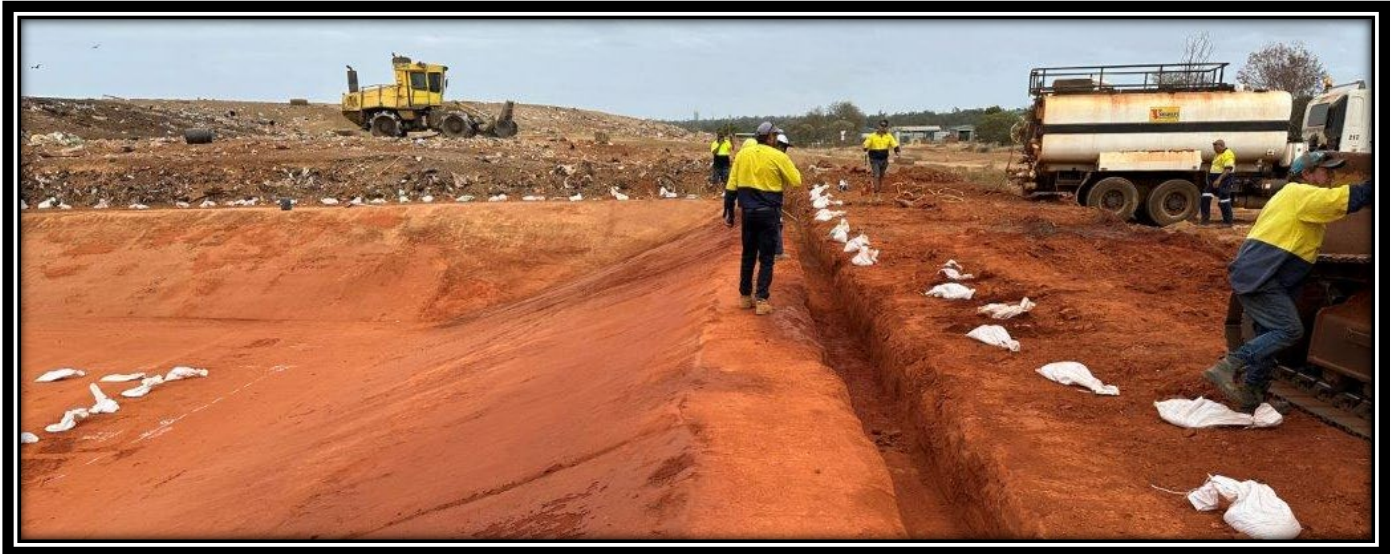
Image 3: Shaping of the cell banks and trench
