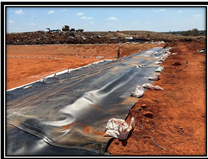
Image 4: Laying Geo-membrane in progress
