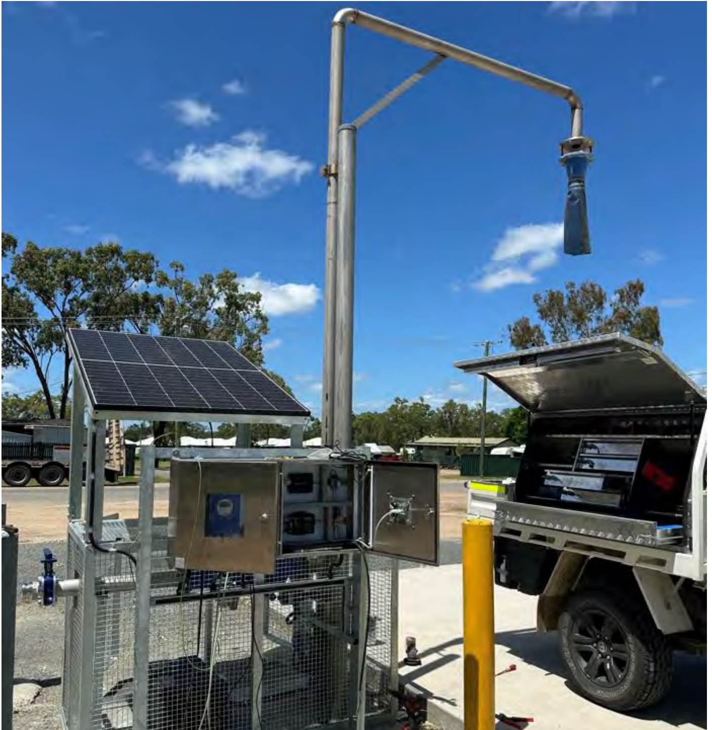
Image 2: Nebo Truck Fill Point –Construction Completed and Commissioned
