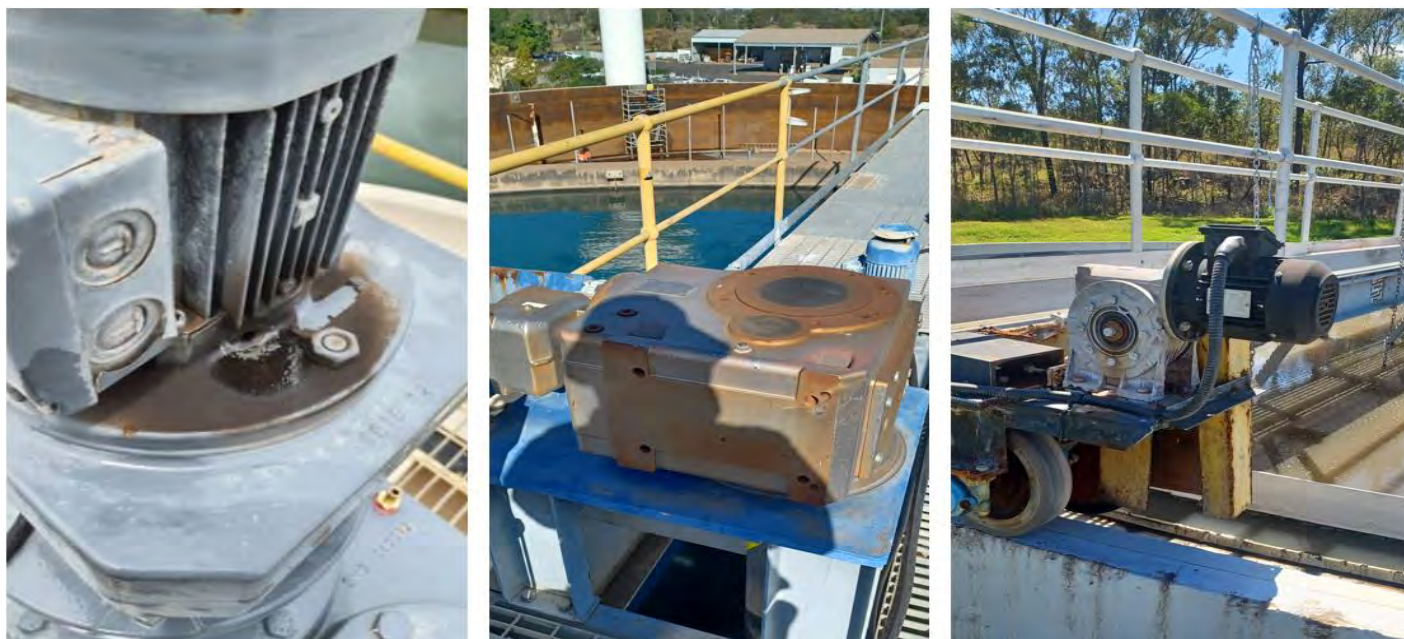
Figure 3 Process equipment maintenance activity
