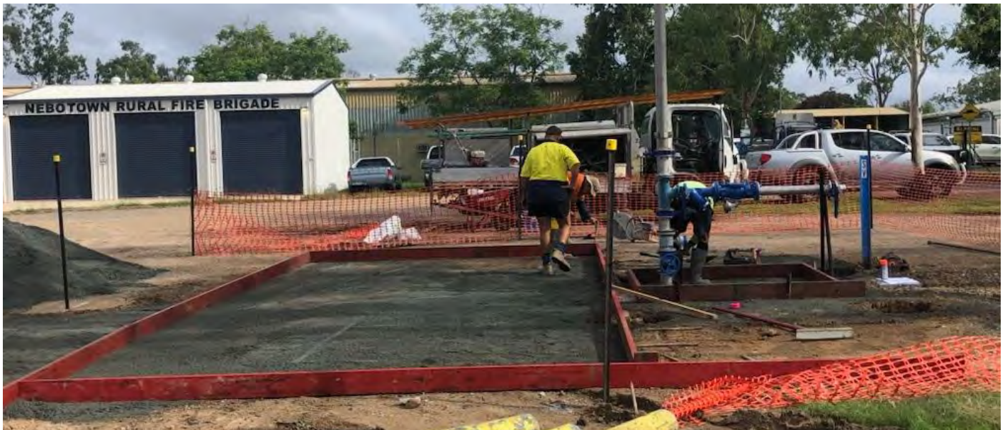
Image 1: Nebo Truck Fill Point – During Construction
