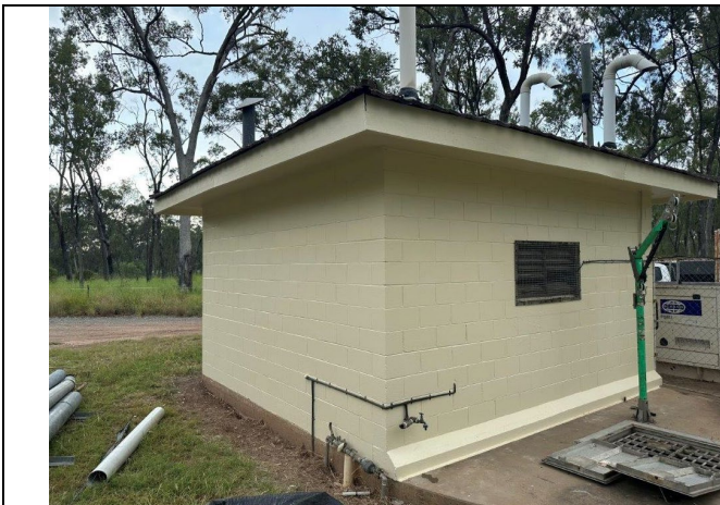
Photo 4 – SPMMT01 building painted
