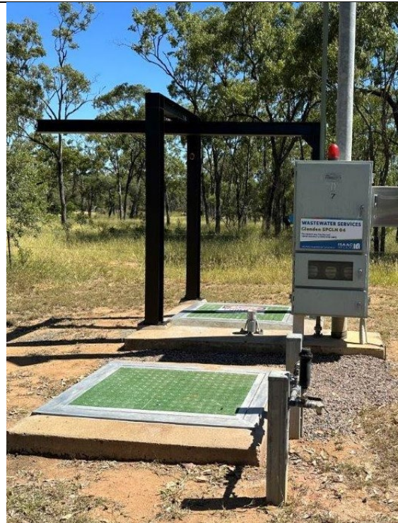
Photo 7 - SPGLN04 – Manholes and gantry
