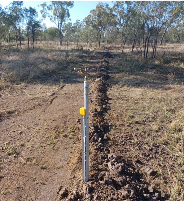
Photo 1 – Riser & Sprinkler
