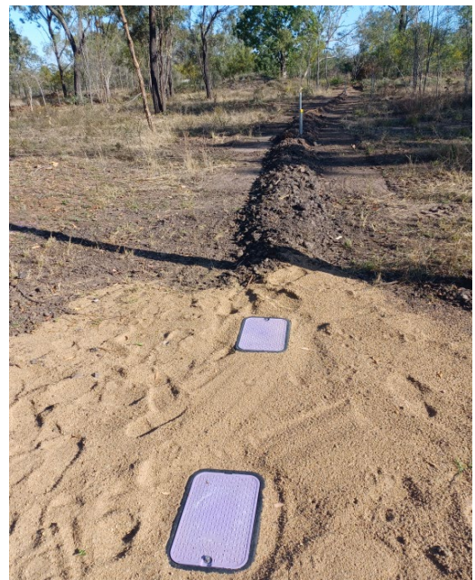
Photo 2 – Sub-surface pipes with manholes
