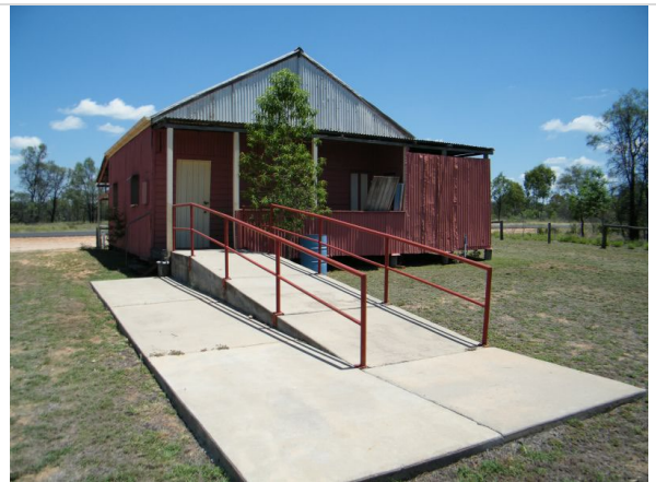
Eastern (rear) elevation showing later concrete ramp addition
