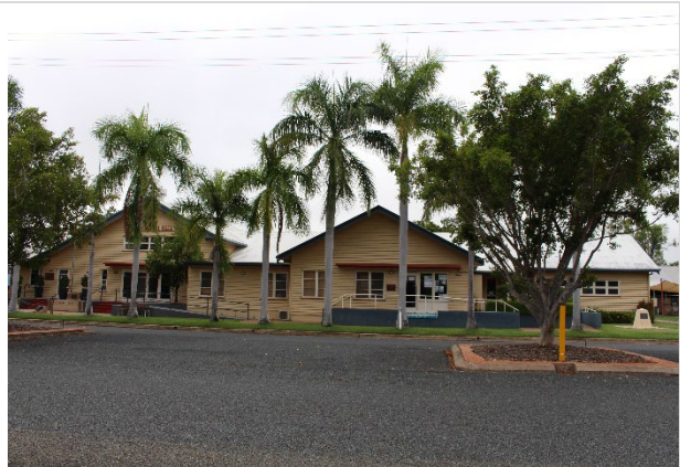
Nebo Memorial Hall and adjoining offices, 2018
