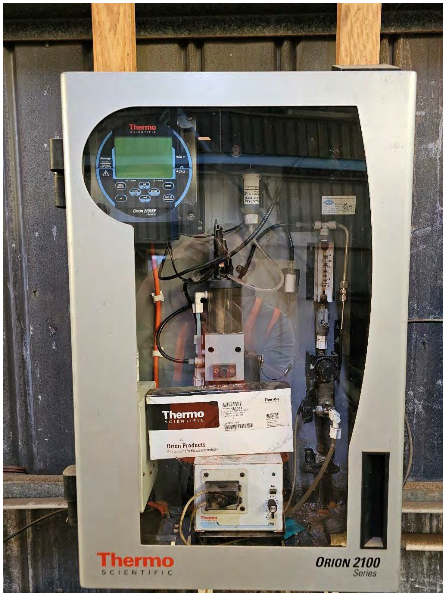
Photo 5: Moranbah WTP Fluoride Analyser (not currently operating)
