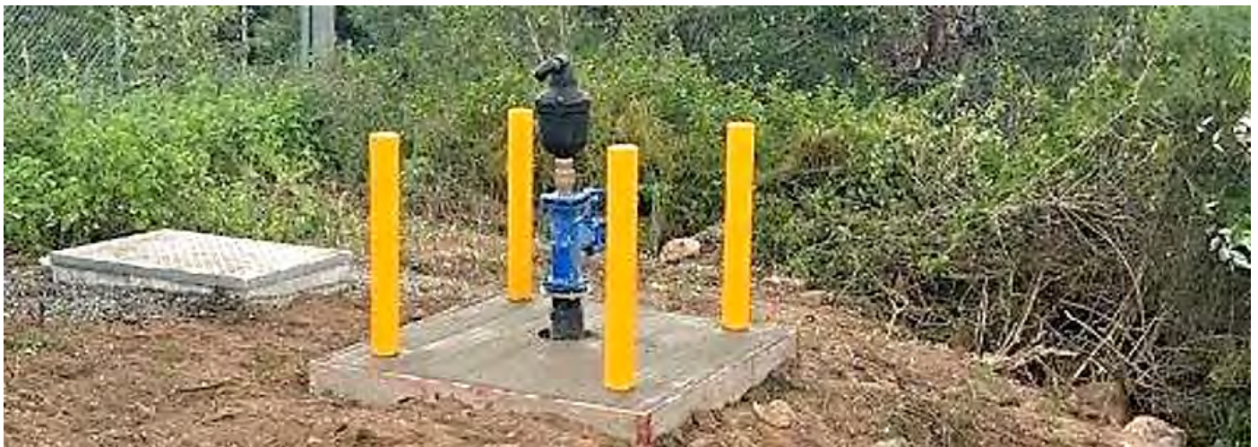
Image 2: St Lawrence Water Storage – New Air Valve installed between Plant and Supply Line
