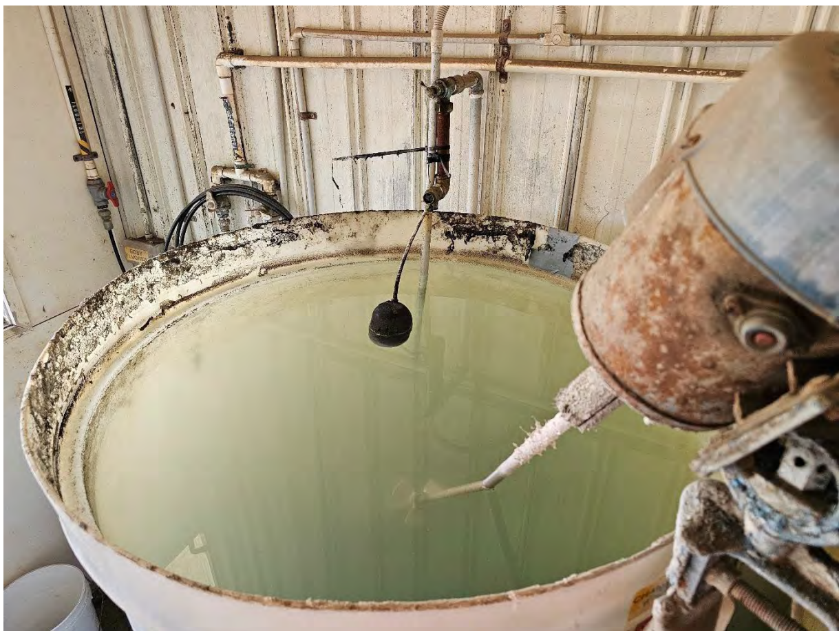
Photo 15: Fluoride Batching Tank Mixer
