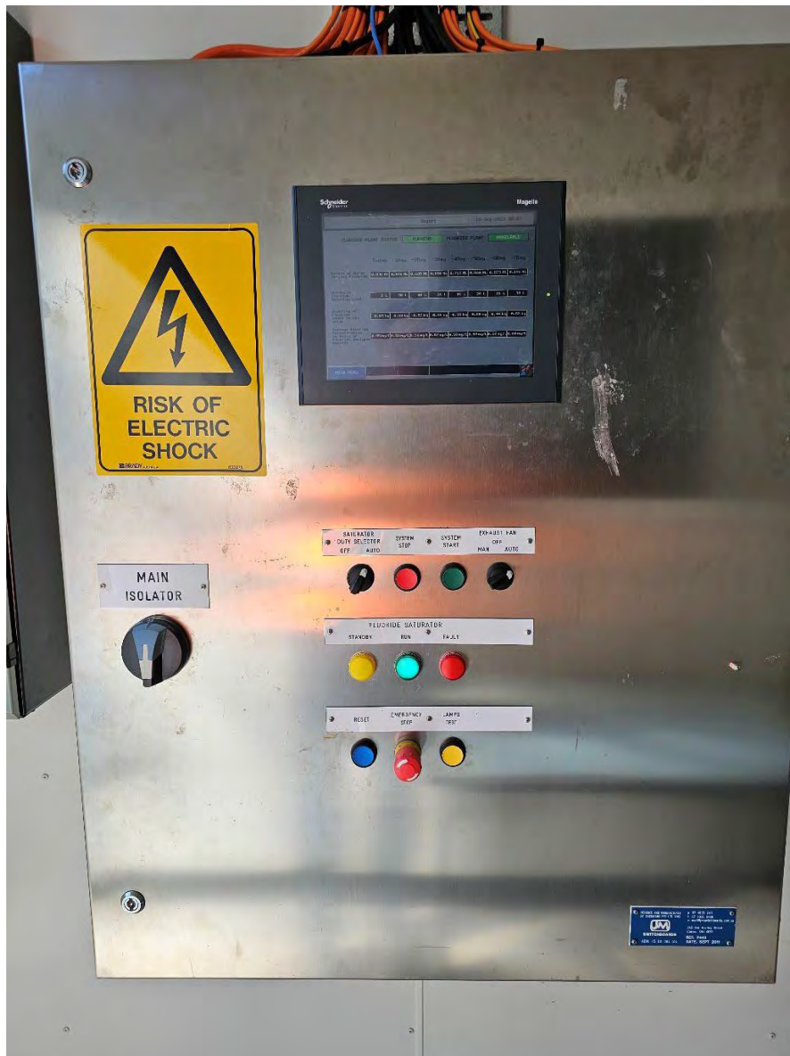
Photo 38: Tieri WTP Fluoride Switchboard Control Panel
