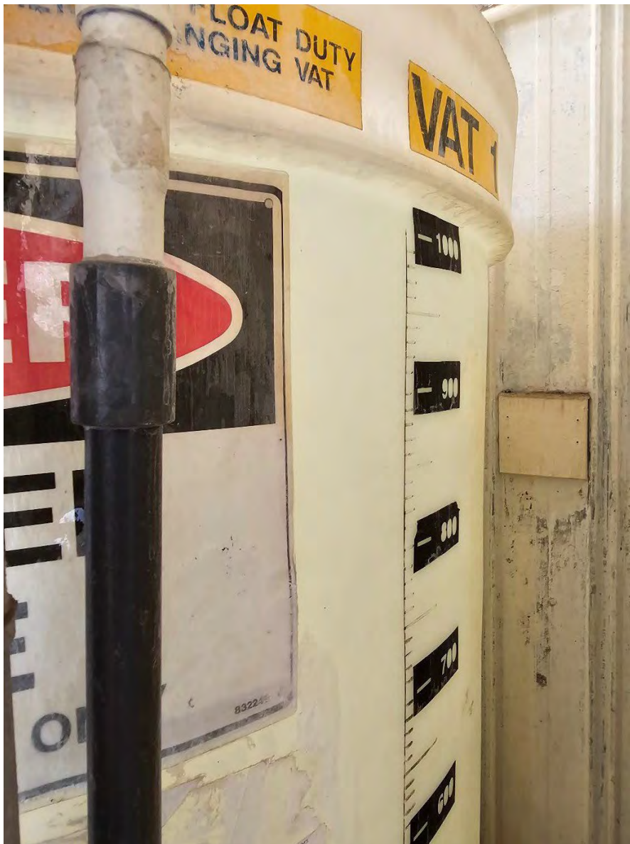
Photo 32: Moranbah WTP Fluoride Dosing System Graduated Lines – Compliant with intent of Code of Practice Item 4.6.12
