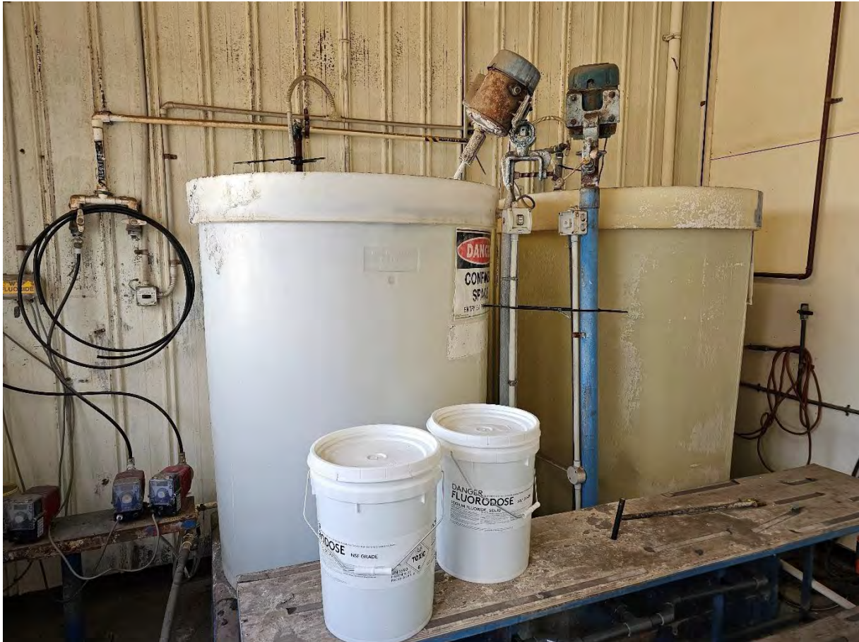
Photo 2: Moranbah WTP Fluoride Batching System
