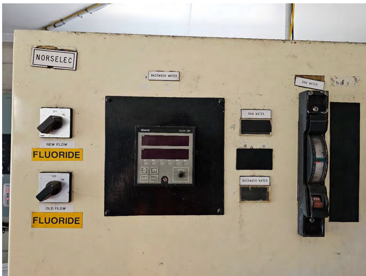
Photo 26: Moranbah WTP Fluoride Control Panel – Compliant with Code of Practice Item 3.3.1
