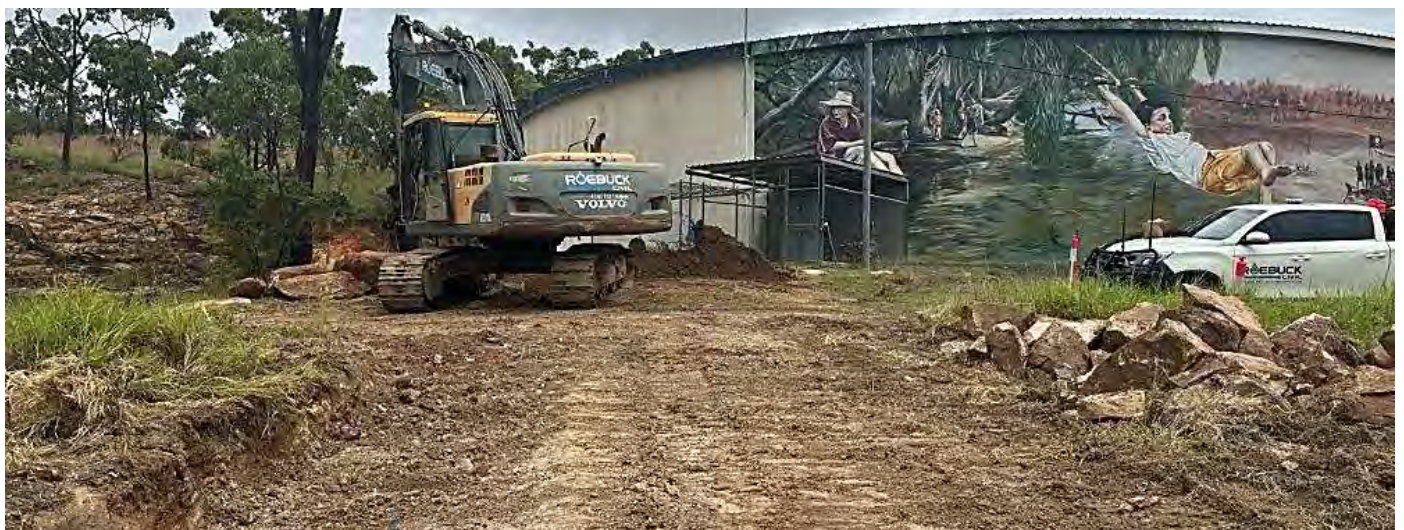
Image 3: Middlemount Water Network Augmentation – Water Main Alignment near Reservoir being cleared
